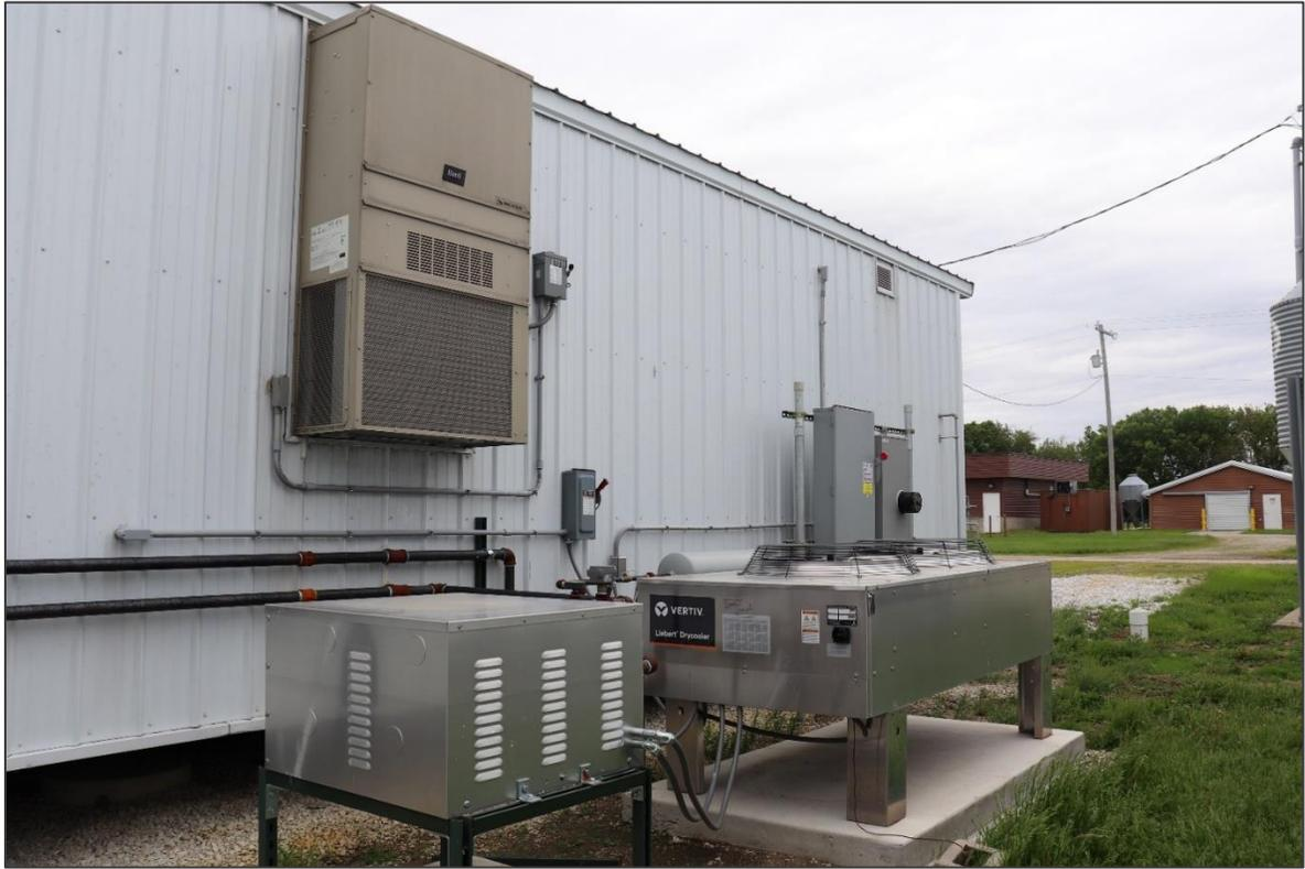
**Figure 3.15.** Dry cooling system.
