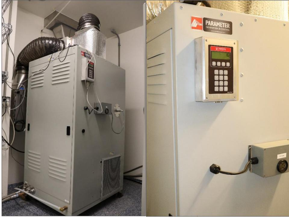
**Figure 3.10.** Parameter Generation and Control (PGC) unit with display.
